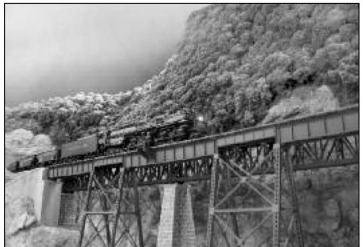
An Allegheny-class leads a coal train over an impressive steel trestle. PHOTO BY CHRIS CARFARO
